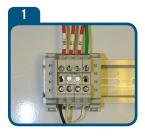
**SET UP:** The first step is to connect your transducer. The data logger is configured to accept standard 2-wire pressure transducers that produce a 4-20mA signal. Connect the + lead to the terminal with wire 10A attached. Connect the – lead to the terminal with wire 20 attached. Connect the shield wire to the terminal with the green ground wire attached.
